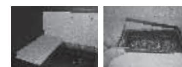
Left side brick 6 positioned on top of left base brick 5. Left mid baffle brick 2 must be held up to enable brick 6 to be fitted. Brick 2 is then supported by left side brick 6.
