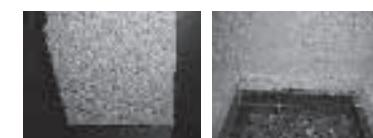
Rear brick 4 positioned lining up tertiary air holes with angled edge sloping down at rear.
