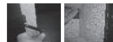
Inner top turbulence brick 1 is positioned on the secondary air pipe with angled edge at rear, sloping down. Brick 1 is held in place with a steel pin.
